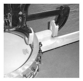
\_\_\_\_\_17. Remove the NECK from the body and clamp it to a sturdy table with your new clamp. Drill a 13/64" pilot hole for the lag bolt. Drill straight to a depth of at least one inch, to match the wood threads of the hanger bolts.
