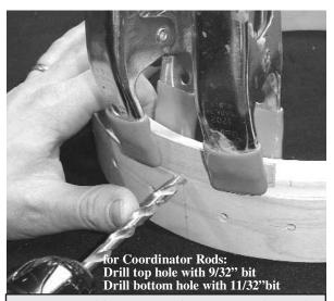
**HINT** - Hold a piece of scrap wood on the inside of the rim where the drill point will poke through to prevent the inside of the RIM from chipping.
