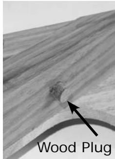
When dry (after an hour or so), you can sand the wood plug flush with the surrounding wood.
